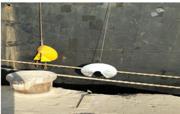
Figure 3. Improper use of rat guard at seaport
