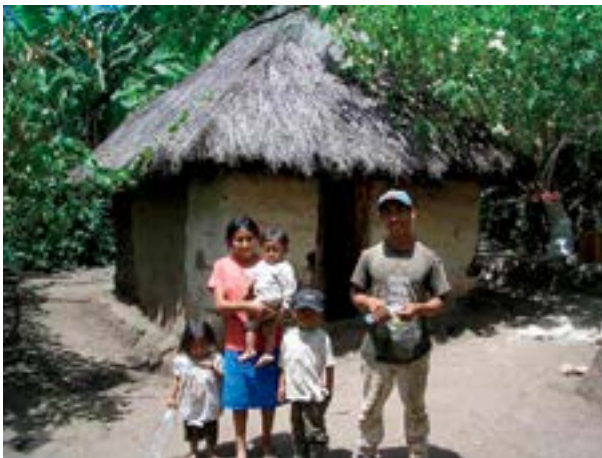
Figure 3 Housing conducive to triatomine infestation. Features such as a thatched roof, dirt floors, and cracked, adobe walls provide ideal habitat for important human vectors of Chagas' disease. (Courtesy of WHO.)
